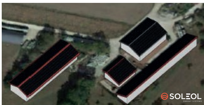
Project in La Chaux Panels 1,545 – Area 2,815 m 2 – Power 564 kW
