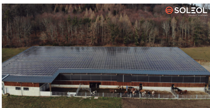
Project in Les Montets Panels 1,704 – Area 2,767 m 2 – Power 528 kW
