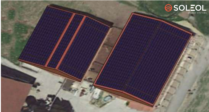
Project in Fontainemelon Panels 1,136 – Area 1,859 m 2 – Power 358 kW
