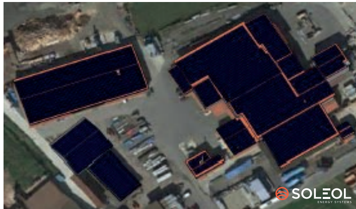
Project in Granges-Veveyse
