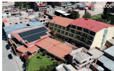
Project in Huaraz Panels 111 - Area 185 m 2 - Power 34 kW
