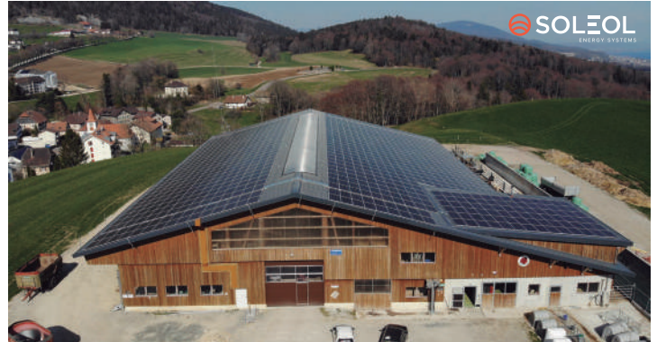
Project in Rochefort Panels 1,104 – Area 1,792 m 2 – Power 342 kW
