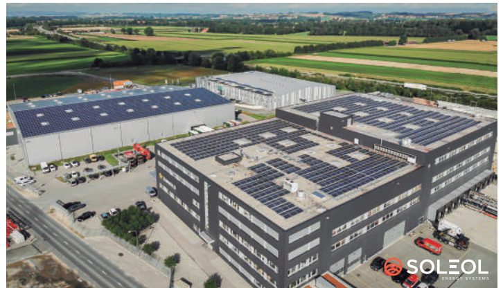
Project in Avenches
