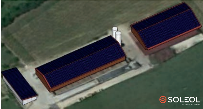
Project in Frégiécourt Panels 1'128 – Area 1,400 m 2 – Power 451 kW
