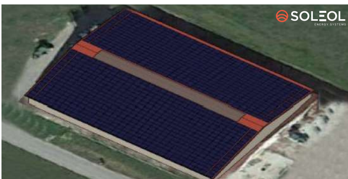
Project in St-Martin Panels 961 – Area 1,803 m 2 – Power 384 kW
