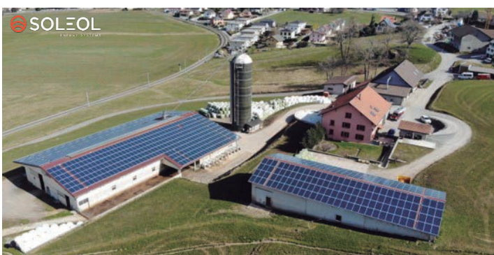
Project in Bossonnens Panels 954 – Area 1,591 m 2 – Power 301 kW
