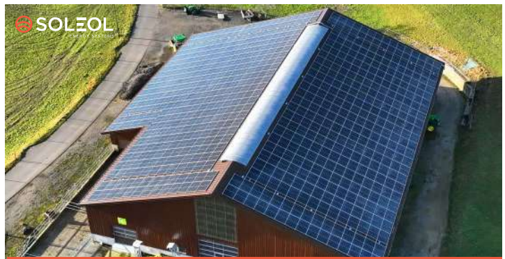
Project in Mézières Panels 558 – Area 1,090 m 2 – Power 229 kW
