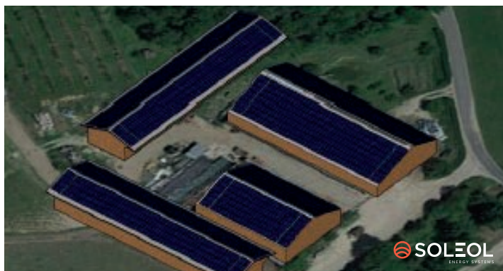
Project in Faoug Panels 1'692 – Area 3'082 m 2 – Power 626 kW
