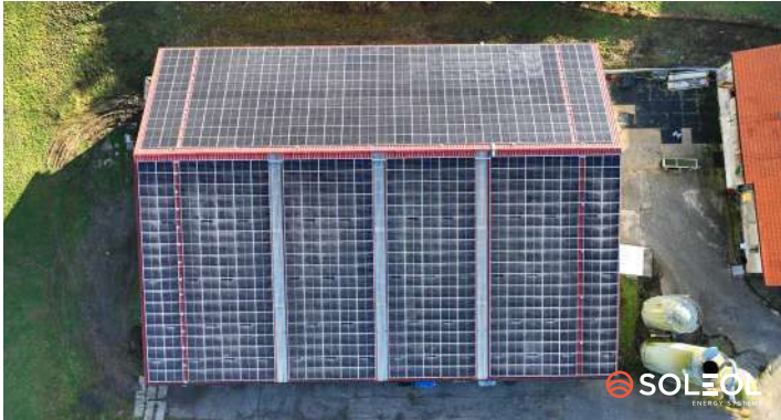
Project in Châtel-St-Denis Panels 742 – Area 1,451 m 2 – Power 304 kW
