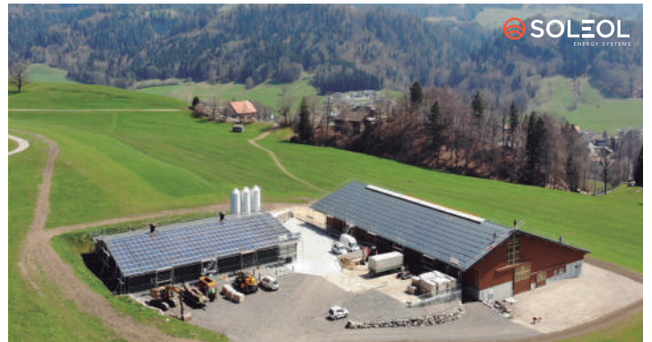
Project in La Roche Panels 1,563 – Area 2,558 m 2 – Power 422 kW
