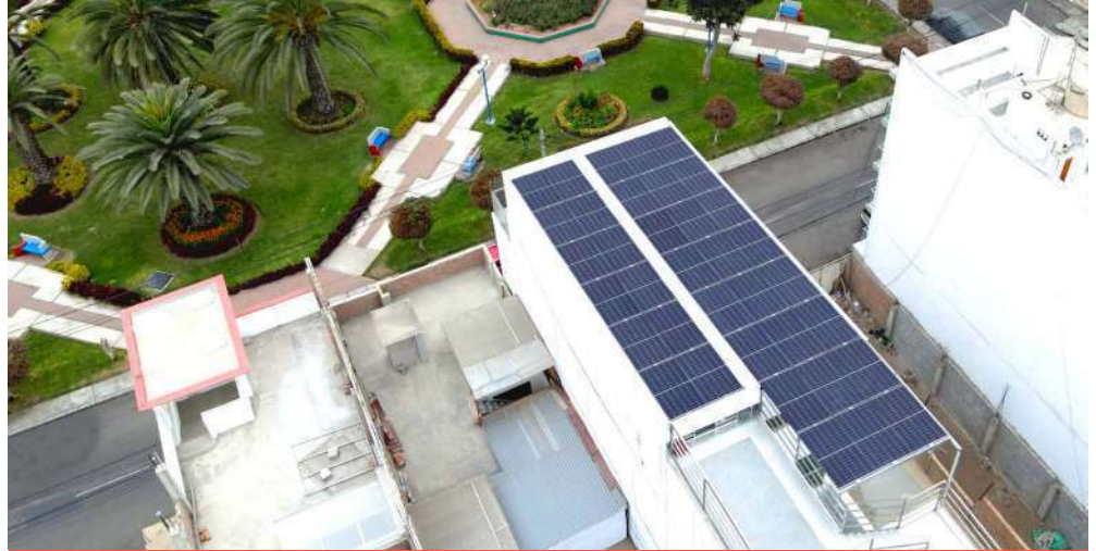
SOLEOL SUIZA BUILDING IN PERU Panels 36 - Area 66 m 2 - Power 13 kW
