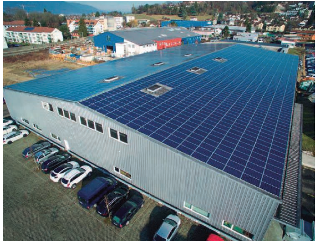
SANPAC IN YVERDON-LES-BAINS
