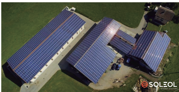
Project in Semsales Panels 1,926 – Area 3,134 m 2 – Power 501 kW
