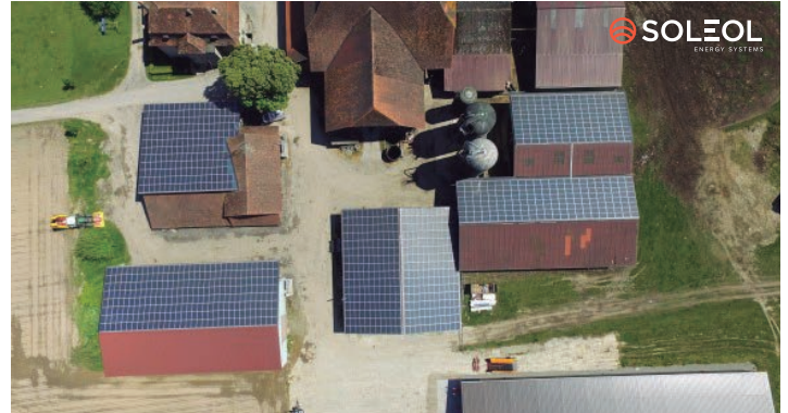
Project in Payerne Panels 1,165 – Area 1,864 m 2 – Power 297 kW
