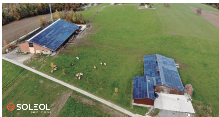
Project in Orzens Panels 1,951 – Area 3,195 m 2 – Power 585 kW
