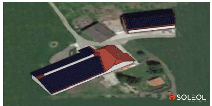
Project in La Brévine NE Panels 788 – Area 1,479 m 2 – Power 307 kW
