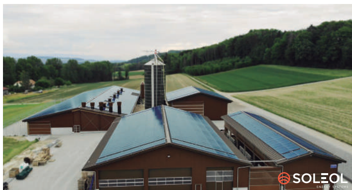
Project in Cudrefin Panels 1'906 – Area 3'184 m 2 – Power 619 kW
