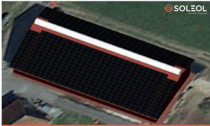
Project in Ecoteaux
