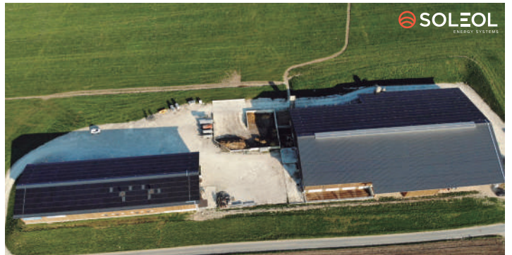
Project in Bournens Panels 1,351 – Area 2,198 m 2 – Power 405 kW
