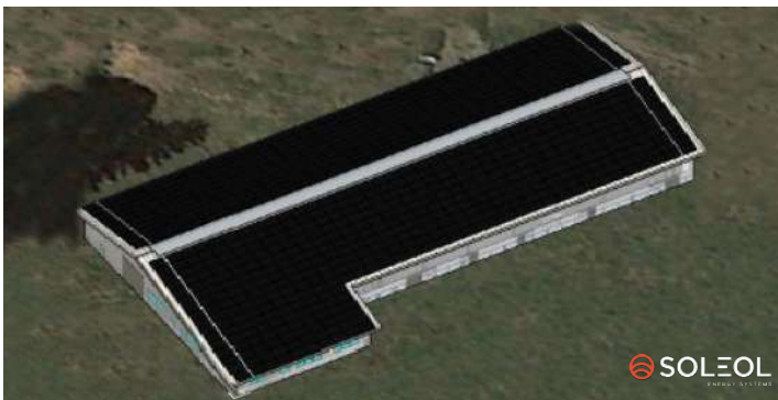
Project in Savigny Panels 790 – Area 1,482 m 2 – Power 308 kW
