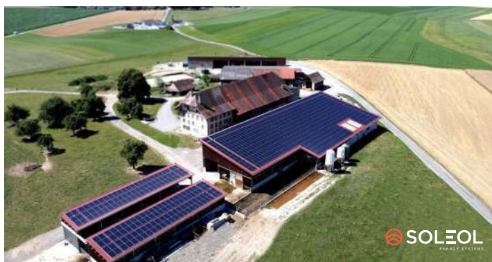
Project in Phontaux Panels 1,481 – Area 2,779 m 2 – Power 592 kW
